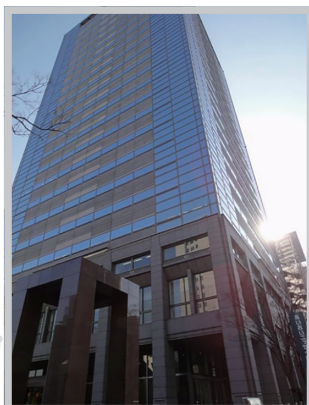
Head Office (本社)
